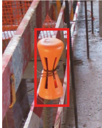
Figure 6. Protected reinforcing rods, where the risk of being impaled is controlled.
