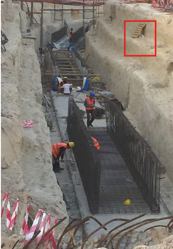
Figure 33. Workers in an excavation.
