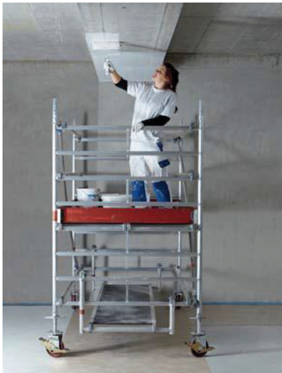
Figure 16. An appropriately constructed mobile scaffold in use.
