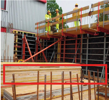
Figure 5. Unprotected reinforcing rods presenting an impaling hazard.
