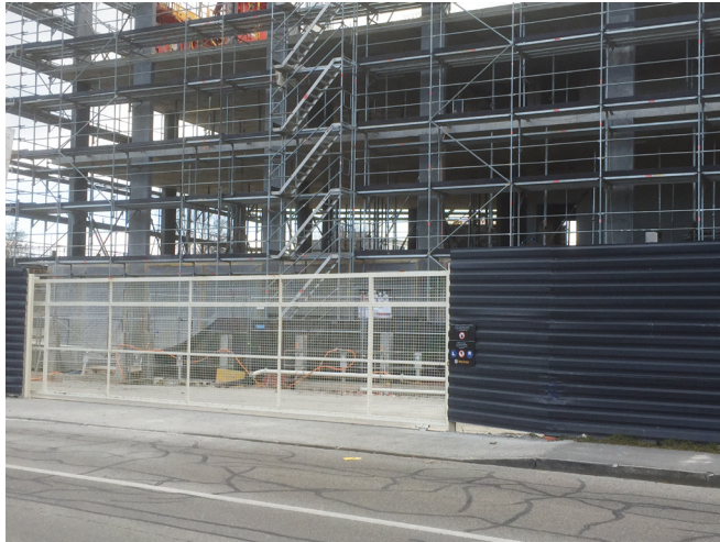
Figure 2. A fenced construction site.
