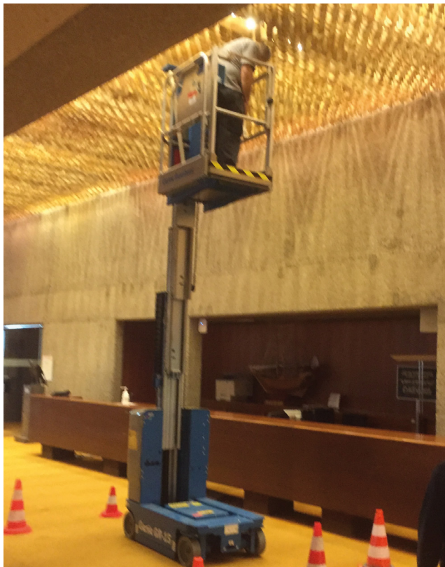
Figure 18. A mobile elevated working platform being used in an office to change light fixtures.
