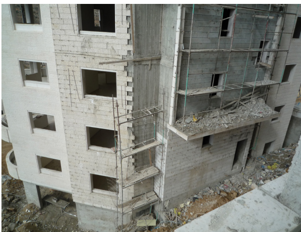
Figure 7. Poor housekeeping depicting debris that could fall onto workers below and an untidy site presenting trip hazards.
