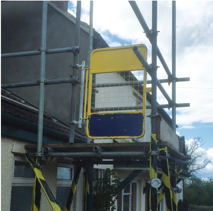
Figure 13. A self-closing gate at a scaffolding access point.
